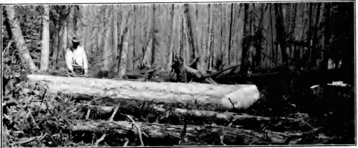
STARTING IN TO EXCAVATE THE HULL.
